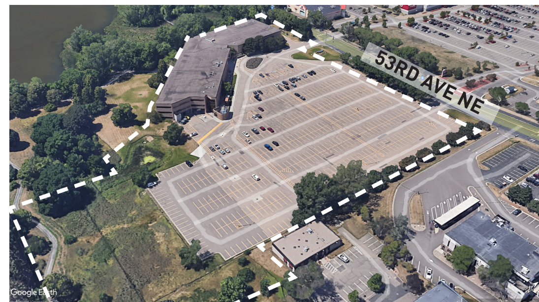
Aerial view looking northwest (Google Earth)
